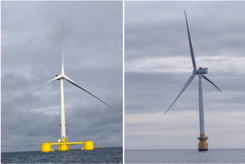
Figure 4. Pictures of floating offshore wind turbine mounted on a semi-submersible platform at Kincardine (left), and on a spar-buoy platform at Hywind Scotland (right).
