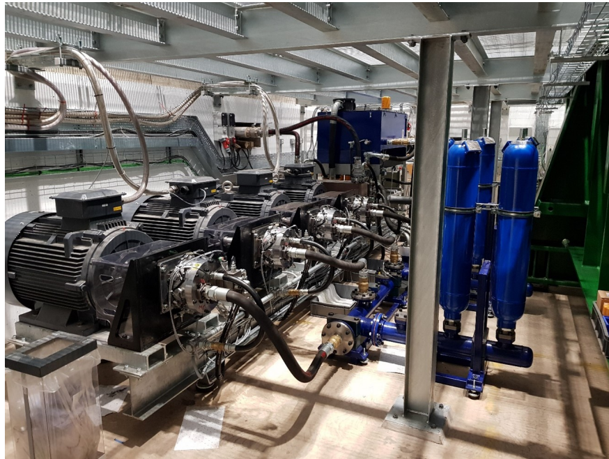
Figure 3.6: Digital Displacement hydraulic pumps during installation in FASTBLADE
