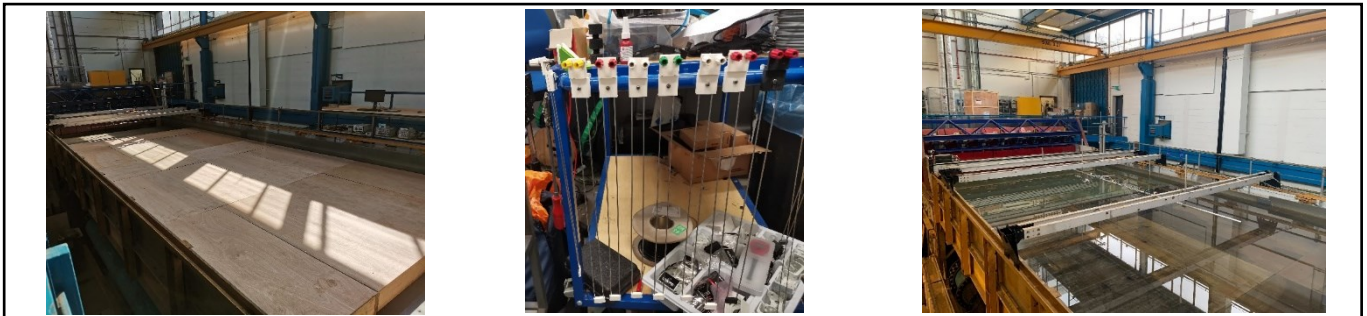
Figure 1: Images of the floor construction (left), new wave gauges (centre) and final experimental set-up (right)
