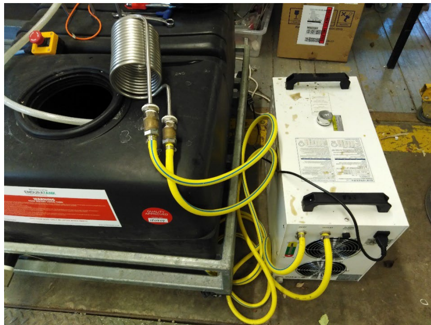
Figure 4b: The chiller with cooling circuit
