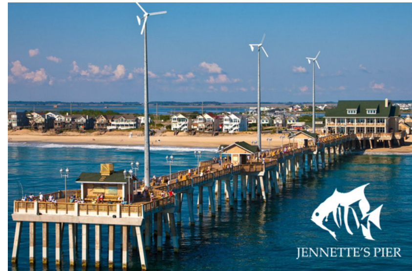
Jennette's Pier, located in North Carolina's Outer Banks, will be the staging ground for the final stage of the Waves to Water Prize.
