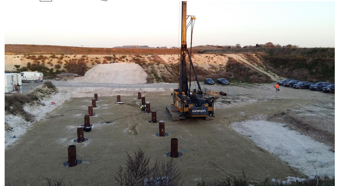
Driving of 508mm OD piles, ALPACA site November 2017
