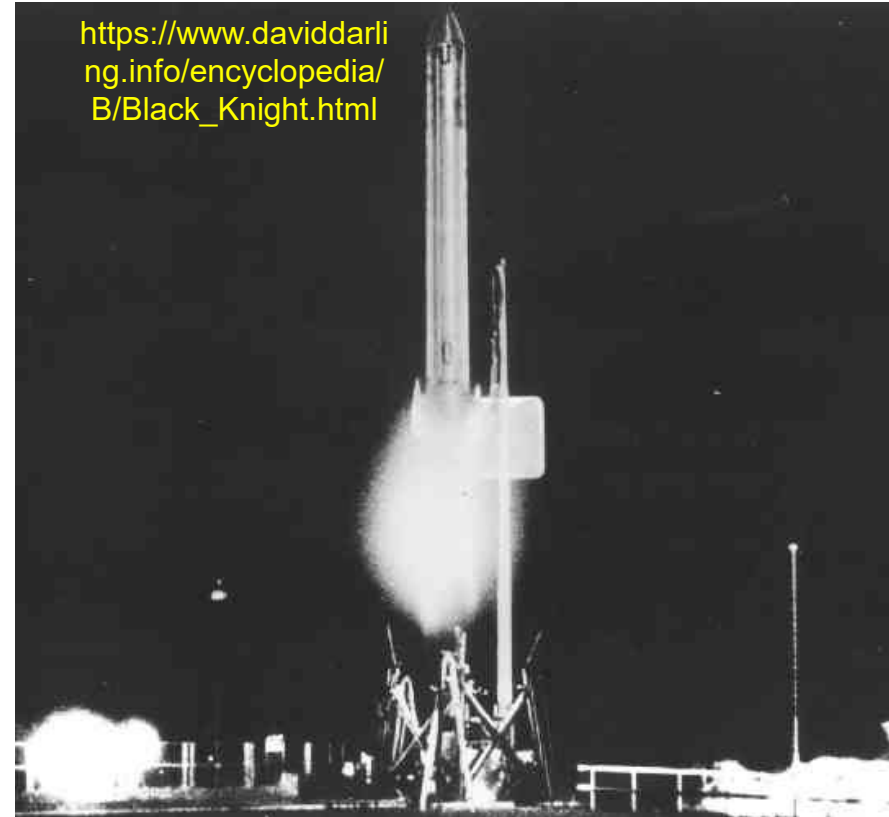
Two-stage version Gaslight Programme 1961-5 11.6 m high, 6.35 tons
