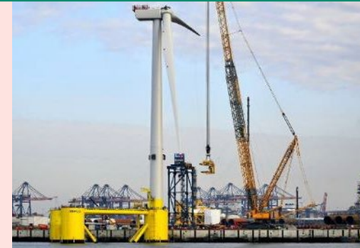
Where the rest of the turbine was attached to the base...
