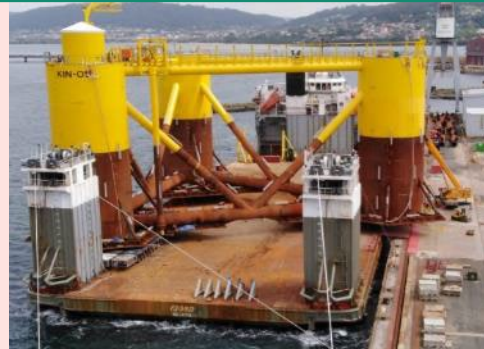
They were loaded on a barge...
