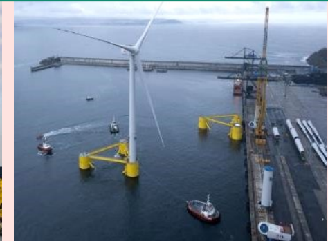
Before being towed out to Scotland
