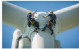
Challenge 3 – Operation & Maintenance and Digitalisation
