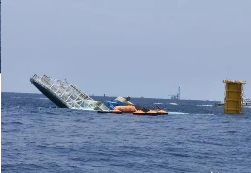
Construction Jack-up Shenping 001, Jul 2021 China
