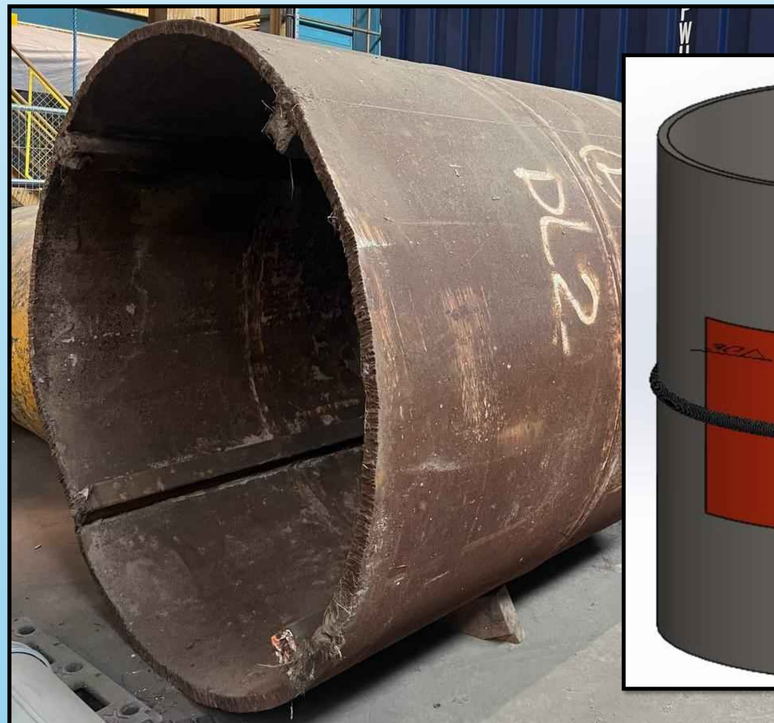
Section of the decommissioned monopile
